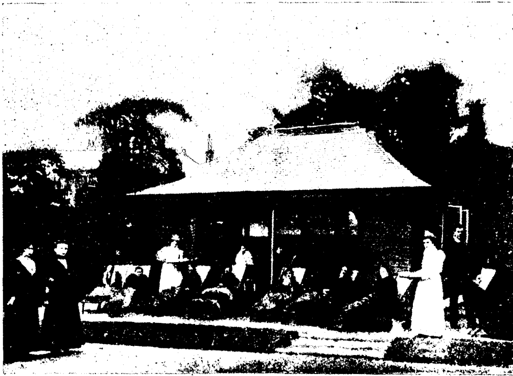
VIEW OF SHELTER HAVING TILED ROOF (Old Pattern).
